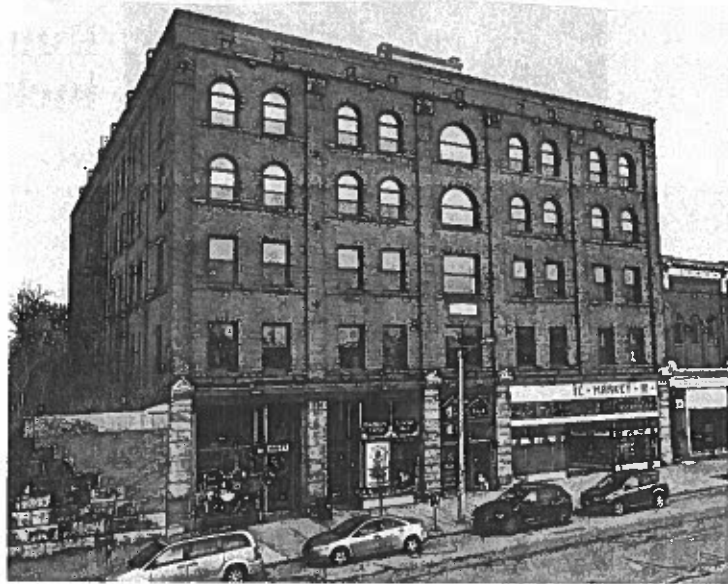
The Mayer Building, 1501-1509 State St., shown here on Jan. 17, 2020, was built in 1899. It is owned by the Performing Artists Collective Alliance and is now home to a theater, art galleries and studios, and more. The building is now listed on the National Register of Historic Places.
