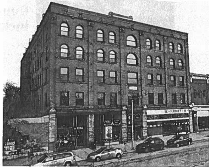
The Mayer Building, 1501-1509 State St., shown here on Jan. 17, 2020, was built in 1899. It is owned by the Performing Artists Collective Alliance and is now home to a theater, art galleries and studios, and more. The building is now listed on the National Register of Historic Places.
