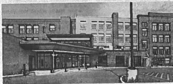
The main entrance to the Erie Center for Arts and Technology is shown on the west side of the former Wayne School in Erie.
