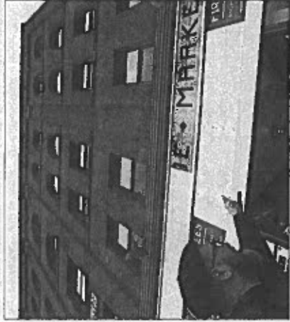
By mid-July, Mark Tanenbaum expects the restored beveled, leaded glass window will be placed in this blank white area in the west facade of the PACA building. (CHRISTOPHER MILLETTE/ERIE TIMES-NEWS)
