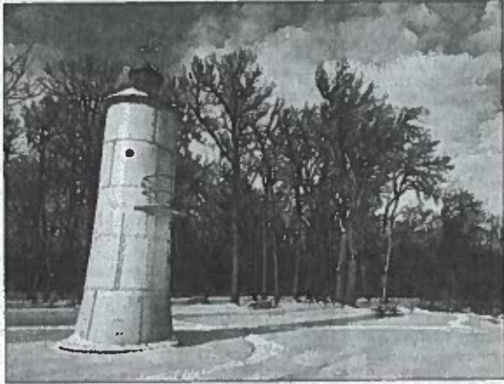
The renovated steel emergency intake gear tower is shown at its new location at Presque Isle State Park on Jan. 29. (PAT BYWATER/ERIE TIMES-NEWS)
