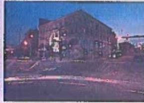
The McGarvey building, located on the southwest corner of 14th and State Streets in Erie, houses Jr.'s Last Laugh Comedy Club on its first floor. FILE PHOTO/DREA WOHLFORD/ERIE TIMES-NEWS
