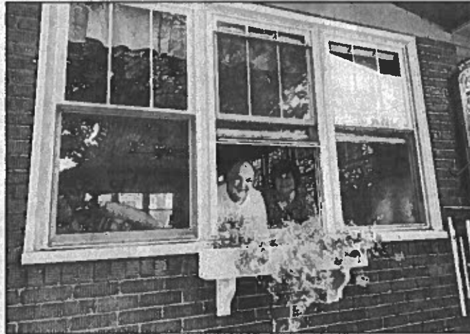
The Browns used grant funds to offset the cost of installing 21 energy-efficient windows in their Corry home.
