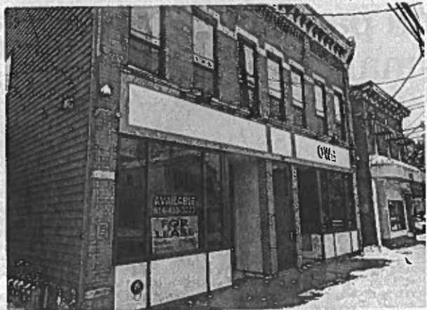
Our West Bayfront's new headquarters in the 400 block of West Eighth Street has been renovated and includes commercial/retail space and three second-floor apartments. KEVIN FLOWERS/ERIE TIMES-NEWS
