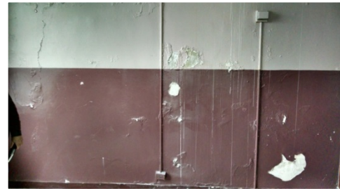
Figure 3: Previous water damage and chipping paint will be repaired and the interior of the hallways and classrooms will be repainted.
