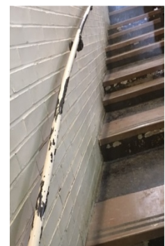
Figure 4: Stairwells will be repaired and repainted.
